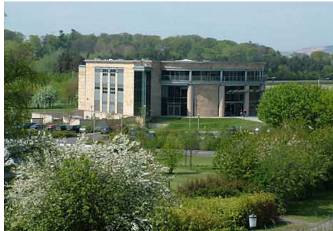
Gateway Building, St Andrews
